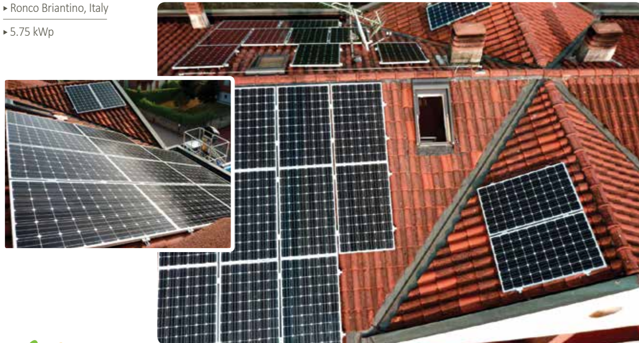
The SolarEdge DC optimized inverter system enabled five additional modules to be installed and only required one 23-module string- despite the roof having asymmetrical and opposite-facing facets.
