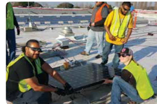
Teamwork to take this roof solar
